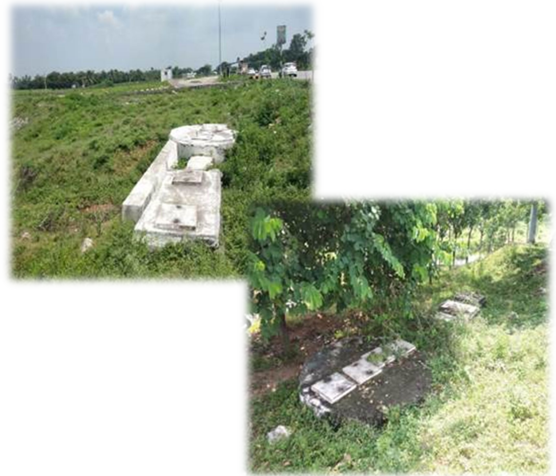
Rainwater Harvesting Structures at toll plaza to conserve water
